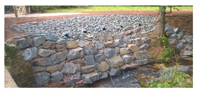
Avenbury Road Bridge is subject to severe flooding from the River Frome. The damage was so severe that the upstream training wall to the bridge was collapsing. The designed solution was to take down the bridge training wall and reconstruct the scoured bank to redirect the flood water back into the river while still protecting the edge of the bridge.
